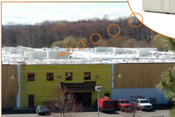
Newington Stew Leonard's During Construction
